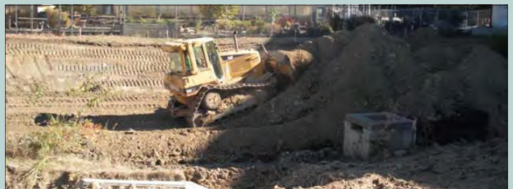
Heavy construction equipment compacts the native soil
