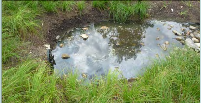
Water ponded in this forebay caused stagnation and conditions amenable for mosquito breeding.
