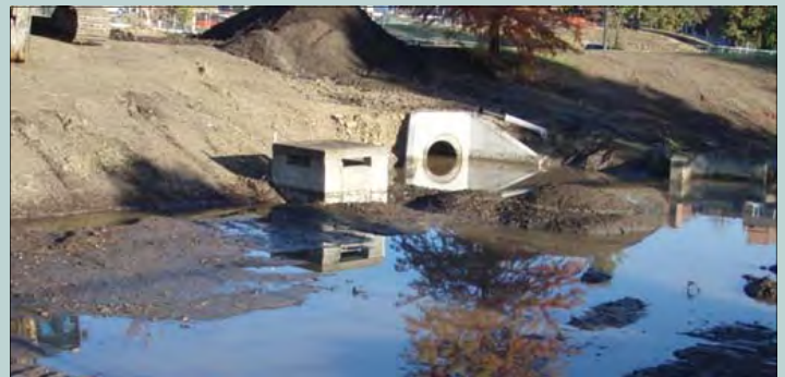
After a rain event, stormwater ponded and sediment built up on top of the bioinfiltration basin's amended soil.
