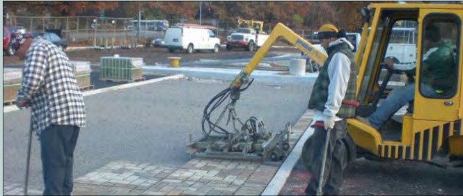
Mechanical paver installation machine provides quick installations of large porous paver systems.
