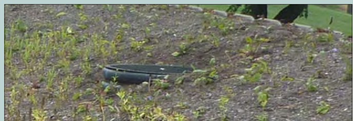
Topsoil can easily wash into this outlet control structure.
