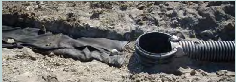
Filter fabric and an underdrain being installed.
