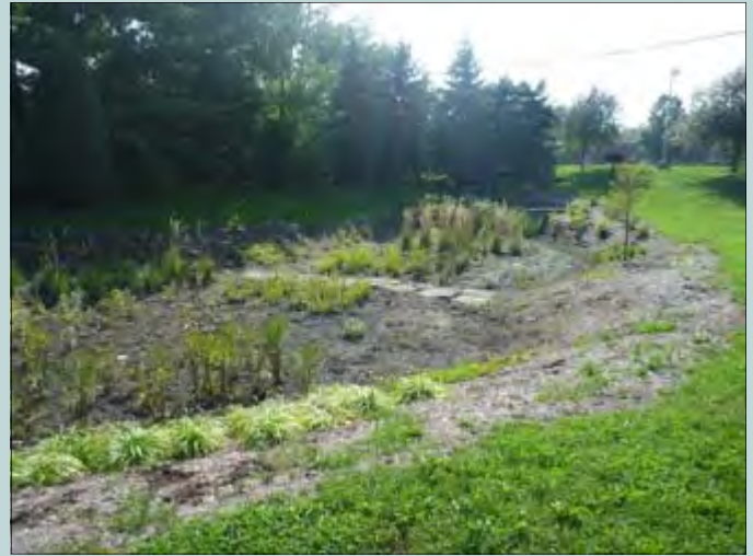
The stormwater has infiltrated through the system 24 hours after the rain event.
