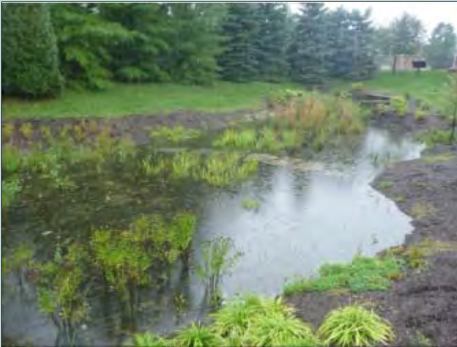
Stormwater ponded in the bioinfiltration basin during a rain event.
